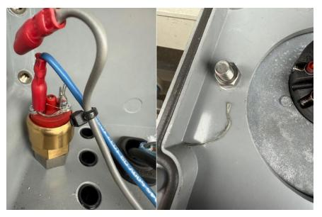
The gray wire has been removed from the terminal for the purposes of taking the photos. But was in place when the bridging wire on the pressure switch was discovered.
